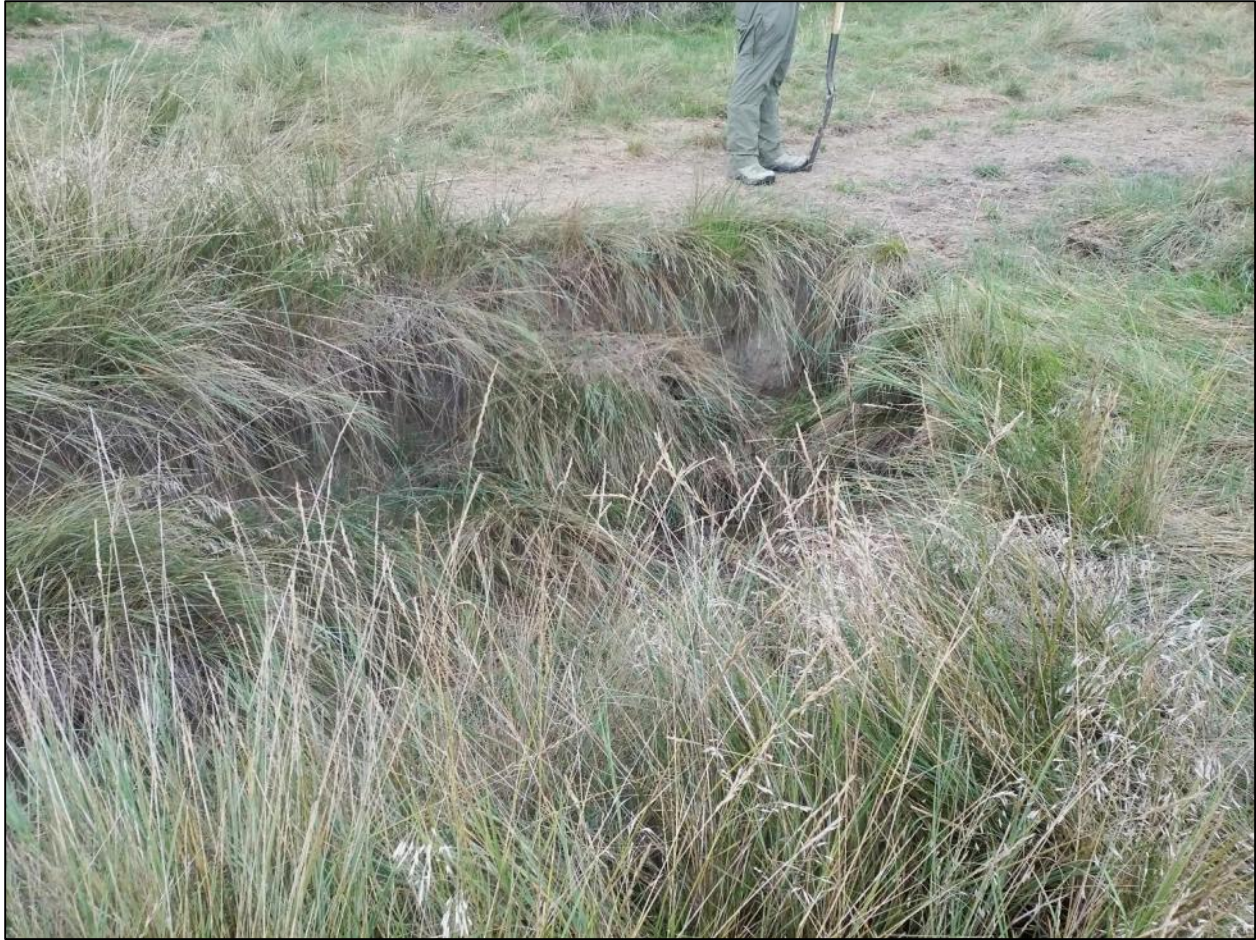
Figure 27. View of 3-4 ft high headcut at upstream end of entrenched channel section 3,000 feet below diversion point.
