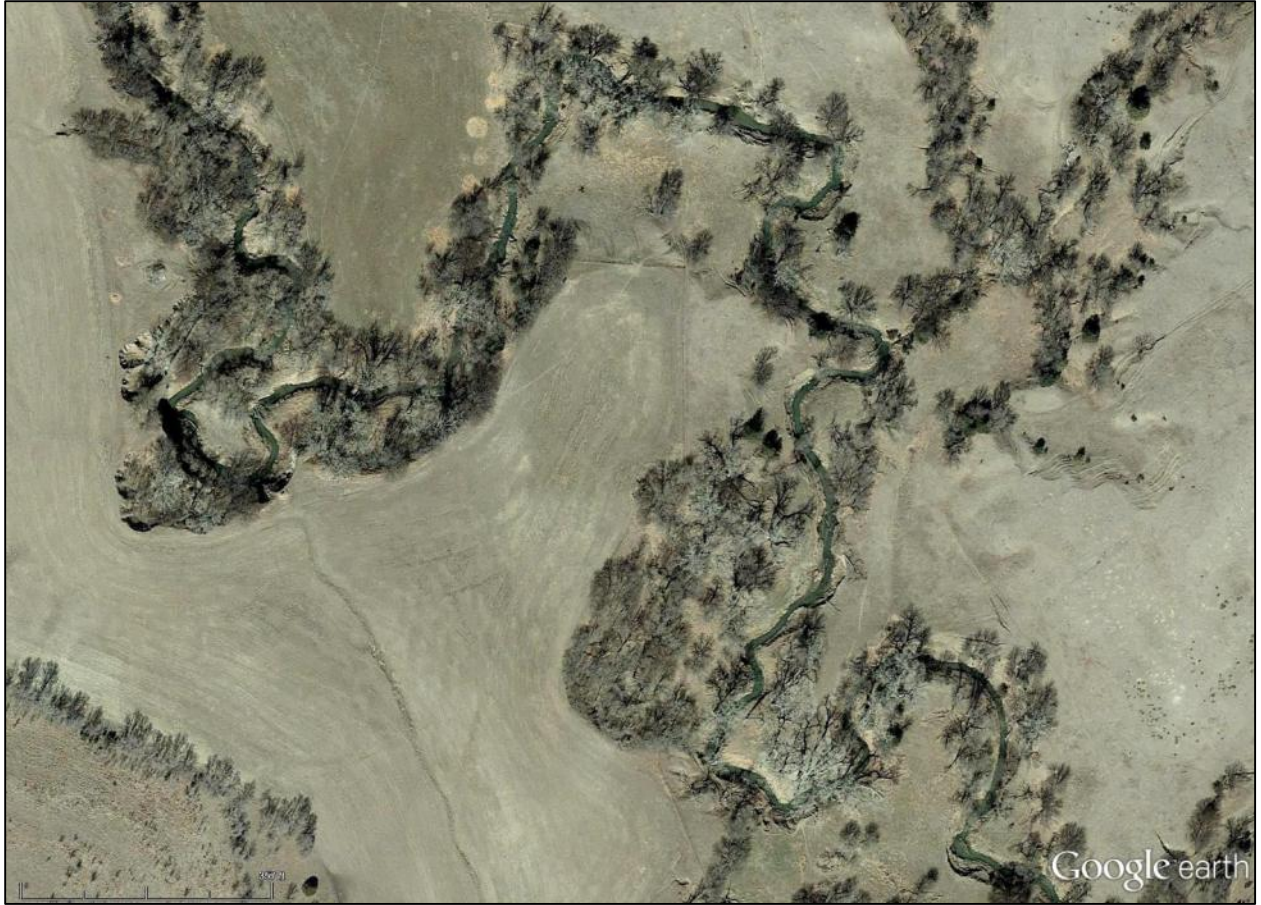
Figure 11. View of tortuous meander bends in the creek between Rd 726 and Rd 727.
