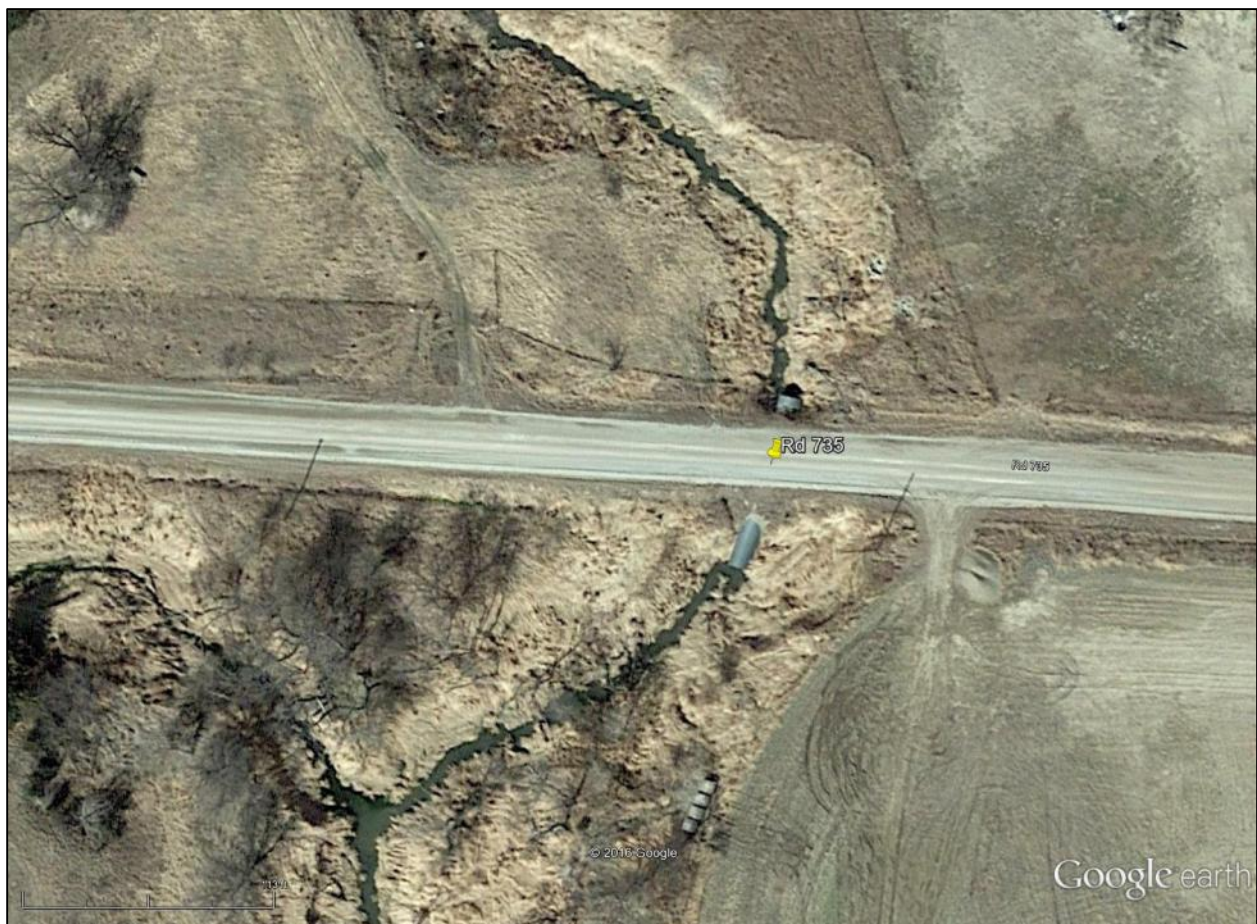
Figure 15. View of the channel and wetlands at the Rd 735 crossing.
