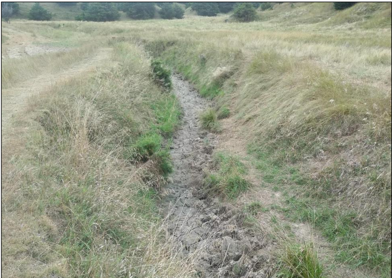
Figure 26. View downstream showing entrenched channel segment about 1 mile downstream of the diversion point. Note shallow gut channel developing in bottom in foreground.
