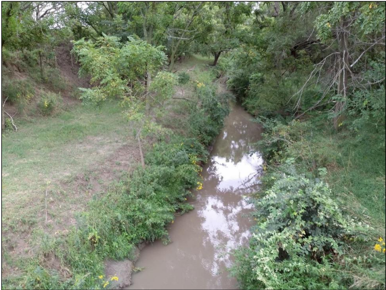
Figure 7. View looking upstream from Rd 720 bridge.
