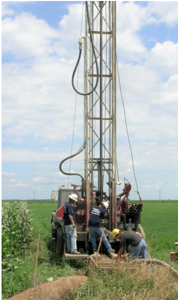
New observation well being drilled in the district.
